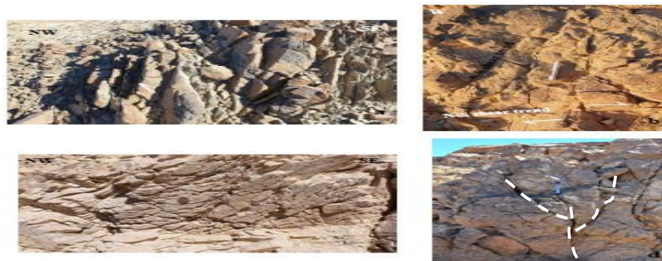
Fig (10) (a) NW-SE shearing in the quartz diorite located west to G.abal Rie El-Garra (b) NS shearing trend dissected by the NE-SW trend in the tonalitic rocks of Semna pluton . (c) Thrust duplex structure in Rie El-Garra syenogranites associating with the NE-SW to ENE-WSW shearing (d) Flower structure accompanying with the E-W shearing in the gneissose granite located at north western part of Rie El-Garra pluton.
